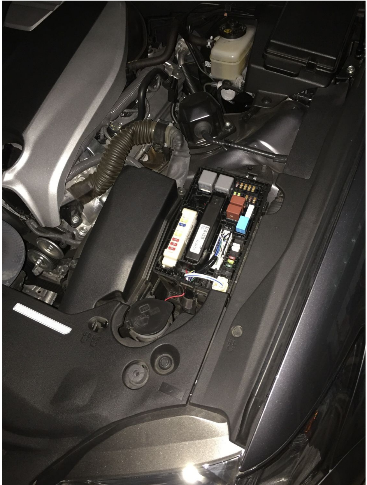
This will be the main wiring harness that you will be tapping
