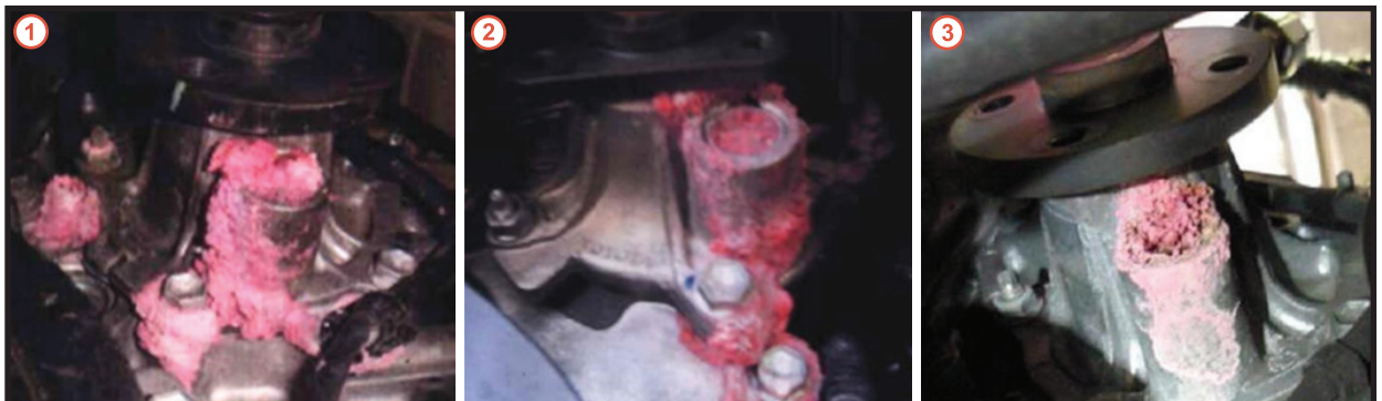
Figure 6. Possible Temporary Leaks – Inspect Water Pump
